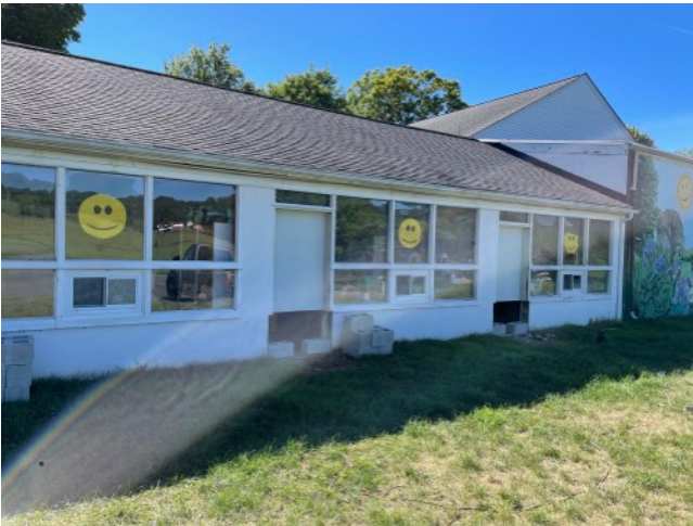
Classrooms with Doors Removed and Old Windows
