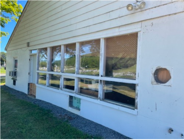
Getz Library with Door Removed and Old Windows
