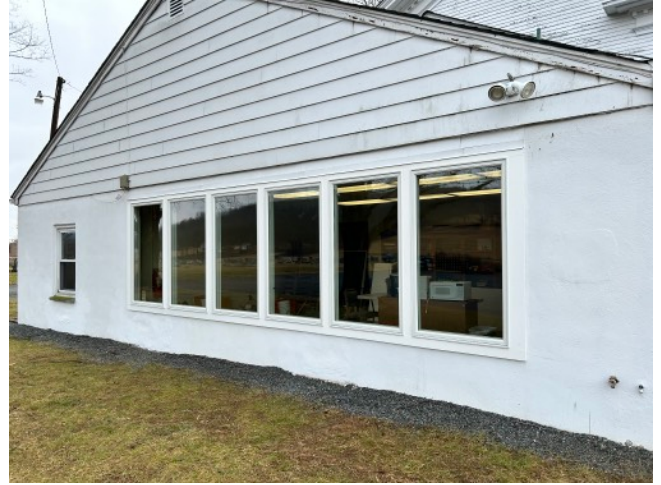
Completed Getz Library Window Replacement
