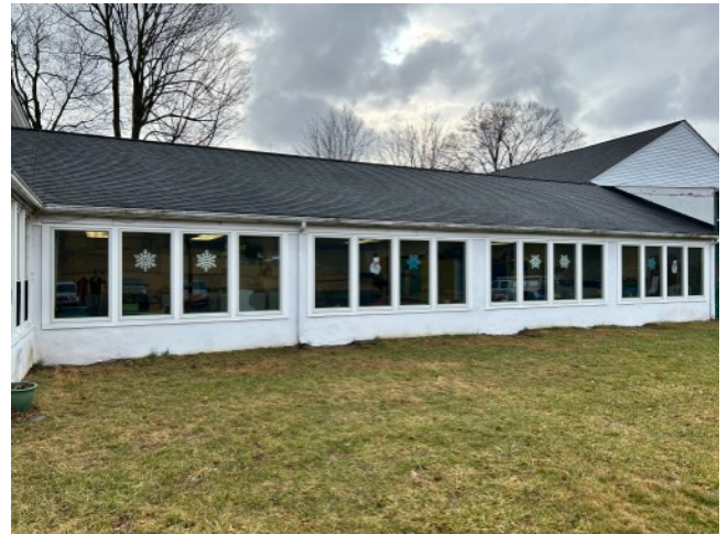
Completed Classroom Window Replacement
